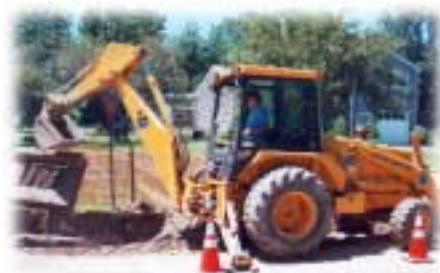
Reconstructing Custer Drive
